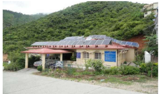
Figure 5 A rooftop solar project at pithoragarh set up by Uttarakhand Renewable Energy Development Agency (Source: The Tribune , 2014)
