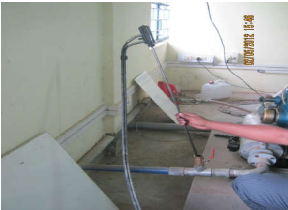
Fig. 2 Flue gas sensor stick inserted into the exhaust valve outlet
