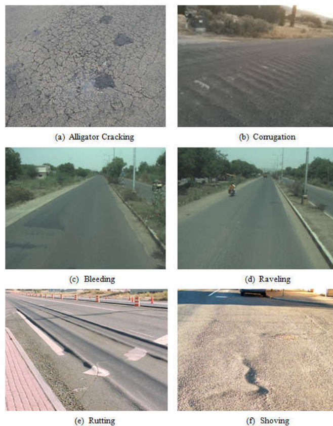
Figure 4 The different distresses of National Highway-752
